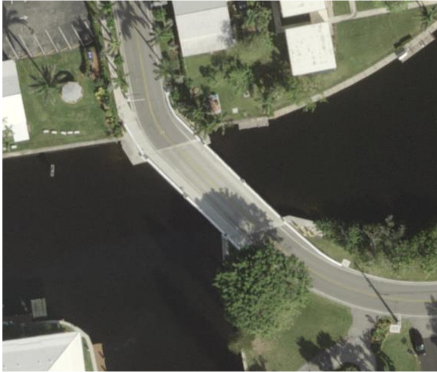
Figure 6 – An example of a feature with culvert characteristics that should be classified as a bridge.
