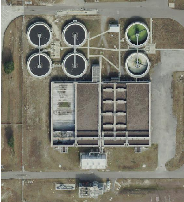
Figure 16- Aerial image of the water treatment facility
