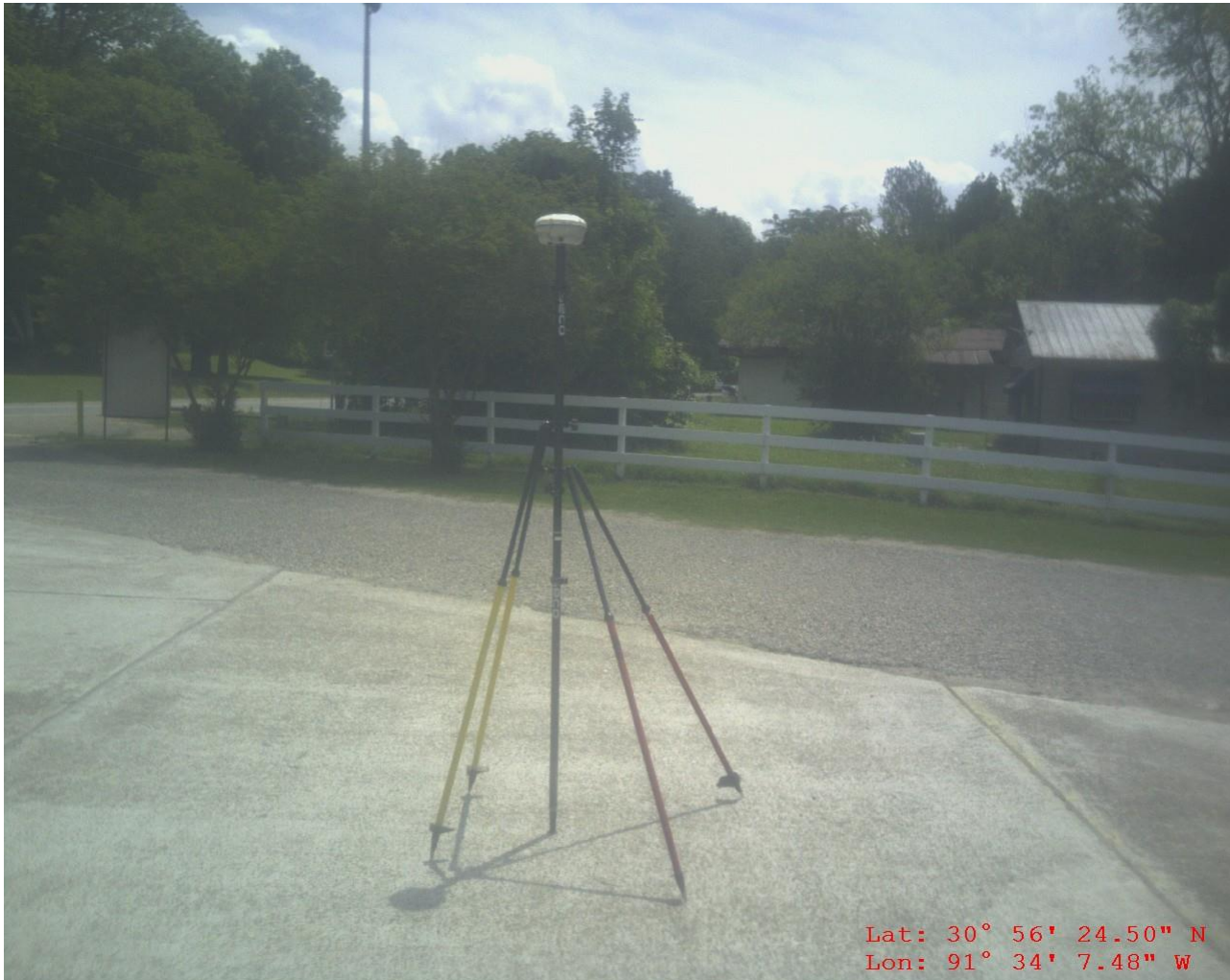
AOI-2 NVA 001 Concrete road
