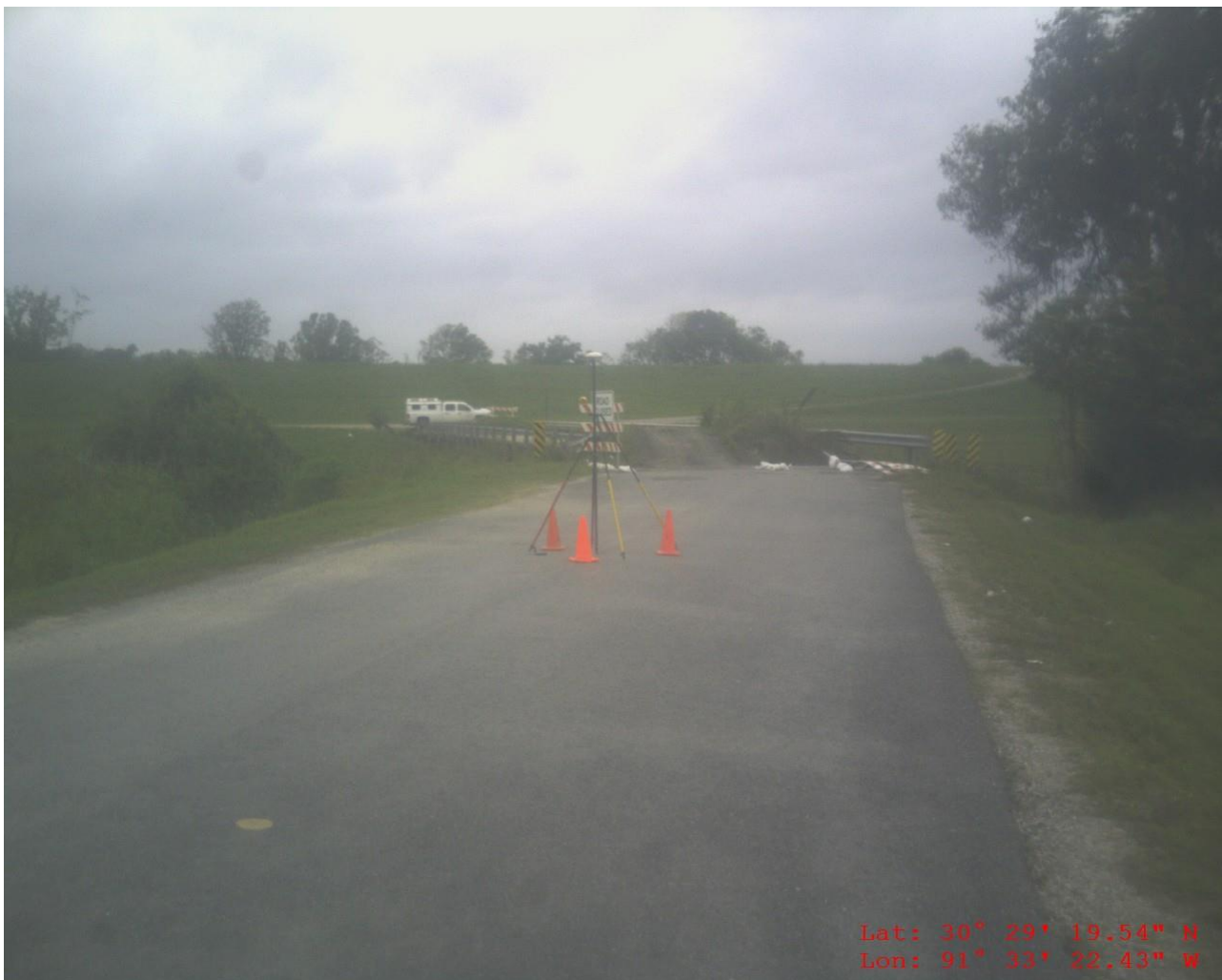
AOI-3 GCP 004 Asphalt road
