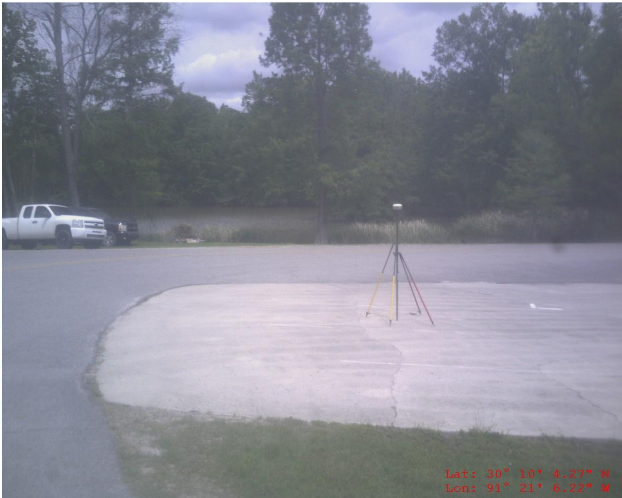
AOI-3 GCP 006 Concrete
