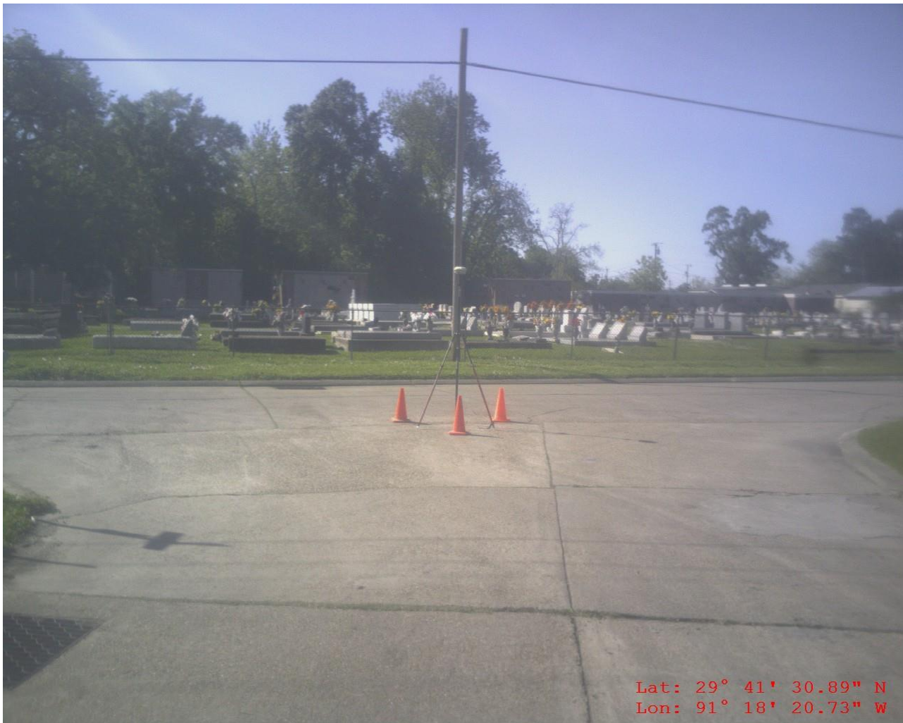
AOI-4 NVA 006 Concrete road
