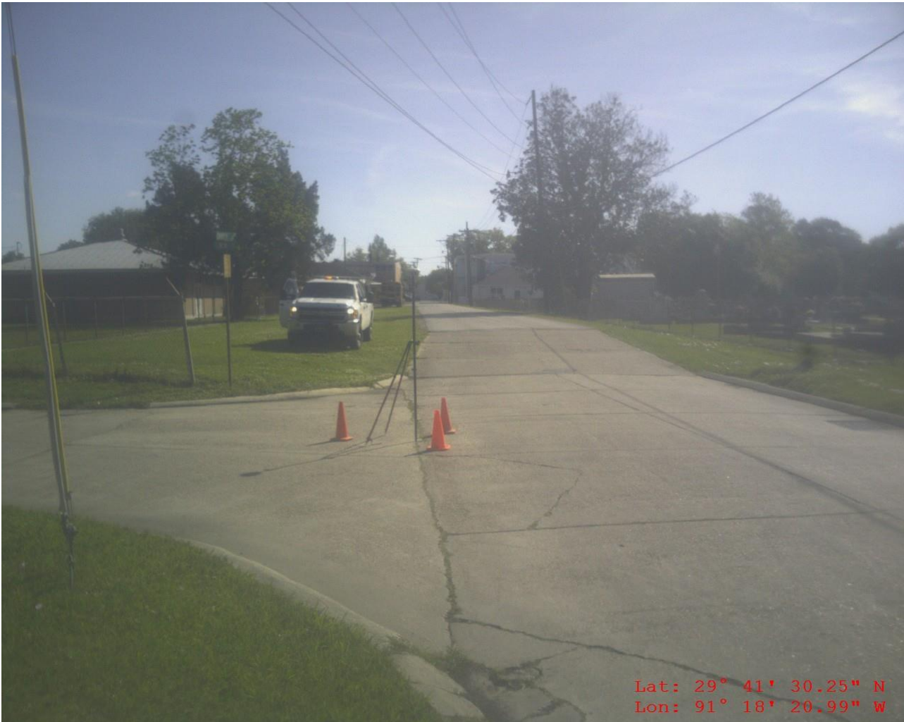
AOI-4 NVA 006 Concrete road
