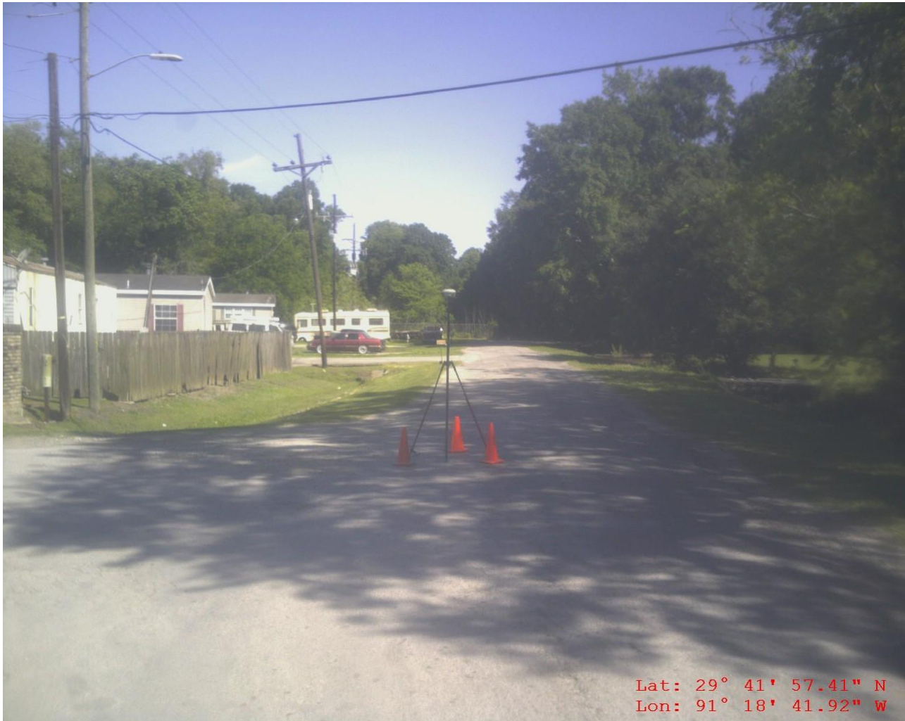
AOI-4 GCP 007 Asphalt road
