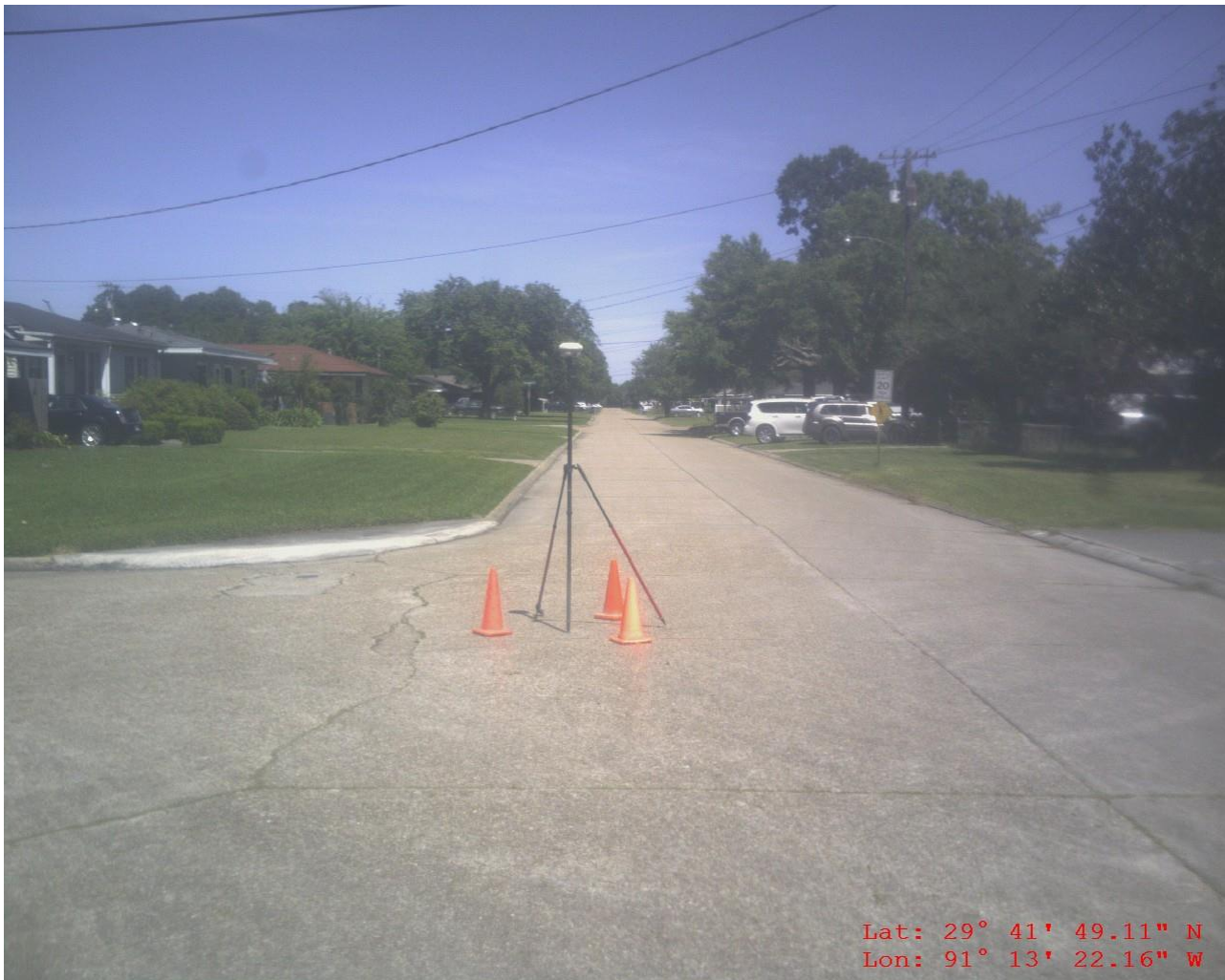
AOI-4 NVA 007 Concrete road
