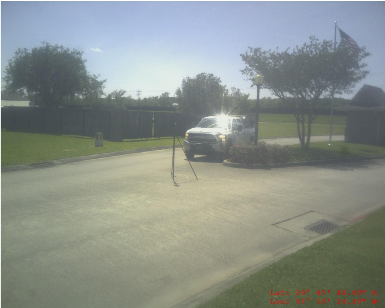
AOI-4 NVA 009 Concrete road
