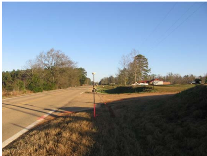
80D NAIL SET 7' EAST OF EAST EDGE OF ASPHALT HWY 541 - 30' SOUTH OF CL OF PAUL CRAFT DRIVE
