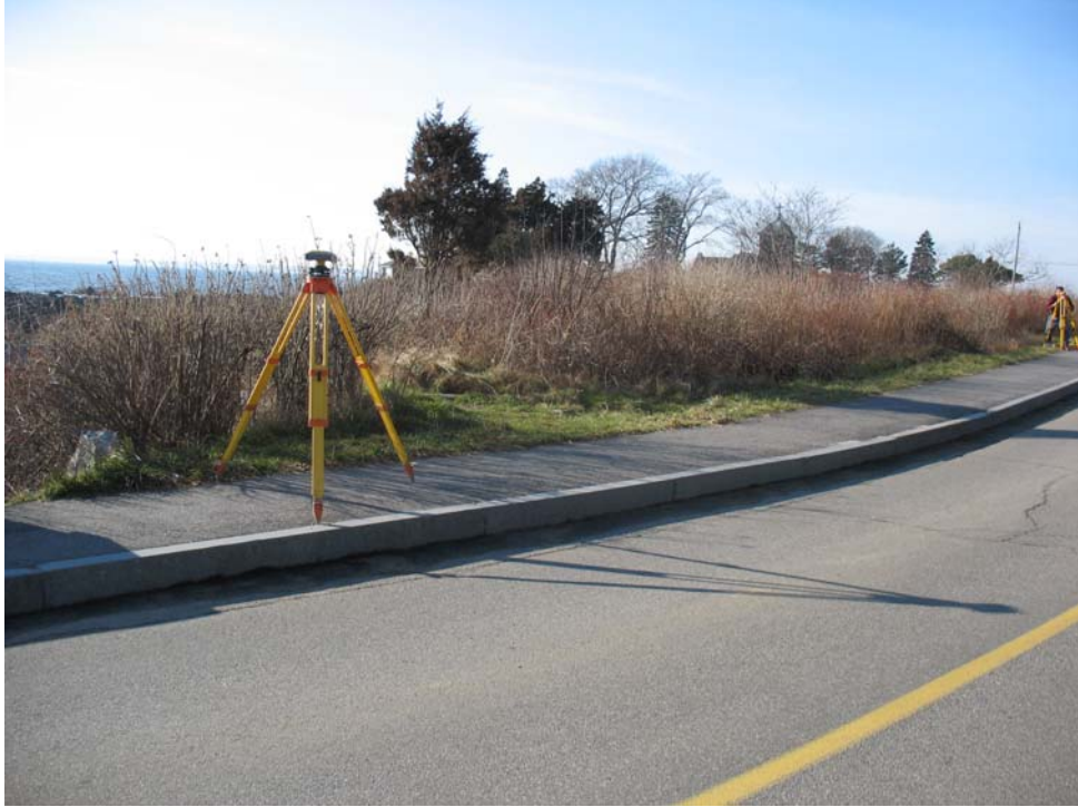
KBP P8 – Pavement
