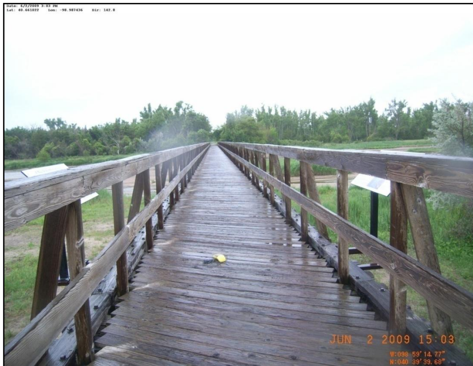
Figure 4: Checkpoint BM-14-8-15C located on a bridge
