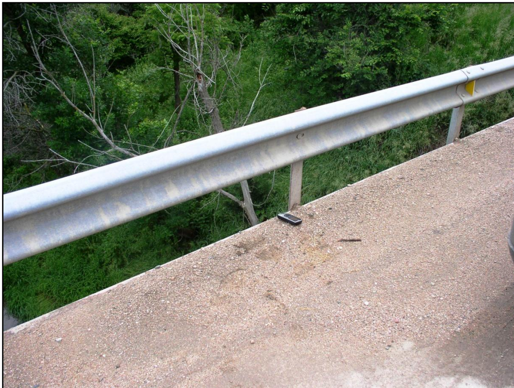
Figure 4: Checkpoint "Spring Cr. Br." located on a bridge
