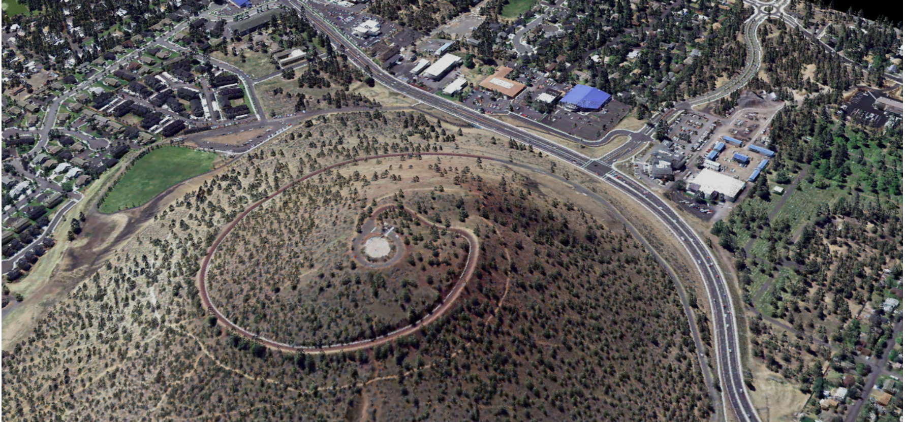
Figure 5.4. View from the Northwest of Pilot Butte near Bend, Oregon. Image is a three dimensional LiDAR point cloud with RGB values extracted from a NAIP orthophoto.
