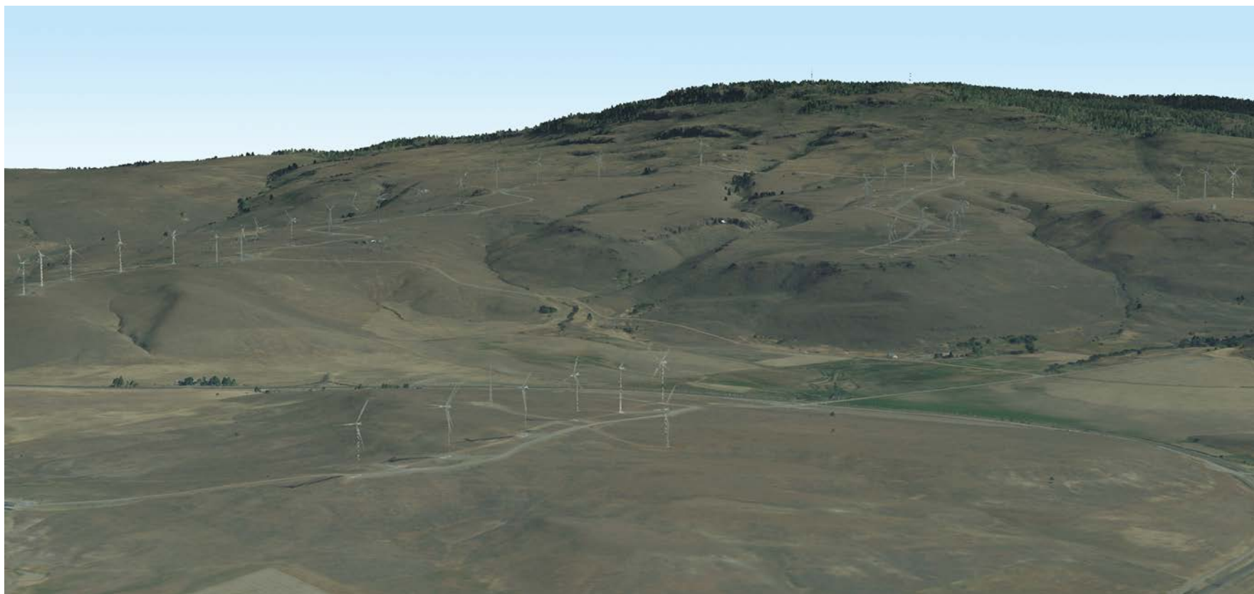
Figure 7.3. Union Baker Area wind farm. Image is a three-dimensional LiDAR point cloud with RGB values extracted from a 2010 NAIP orthophoto.
