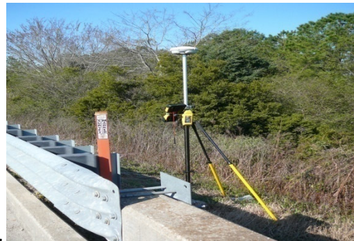
U_8-11-01a – Survey photo– On the bridge
