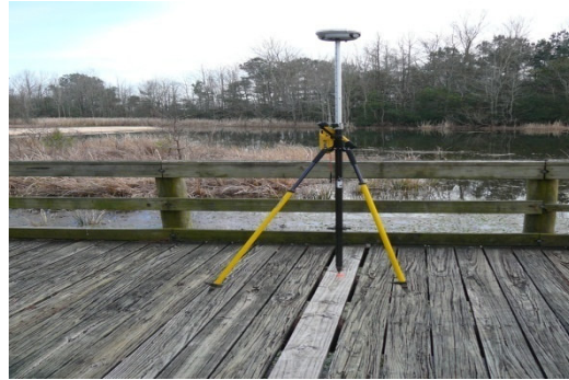
U_8-07-11 – Survey photo– On the bridge
