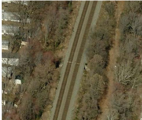
Figure 3 - Bing aerial imagery showing the feature is a culvert.
