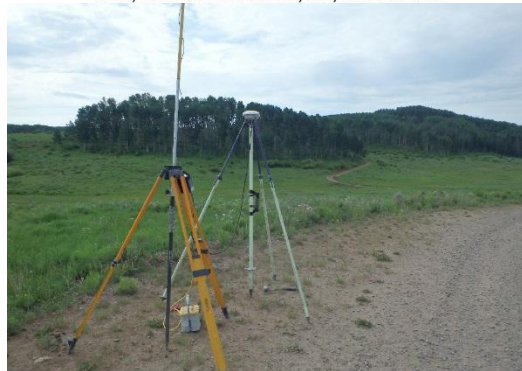
1060, LIDAR CONTROL, 3S, 29JUNE2016
