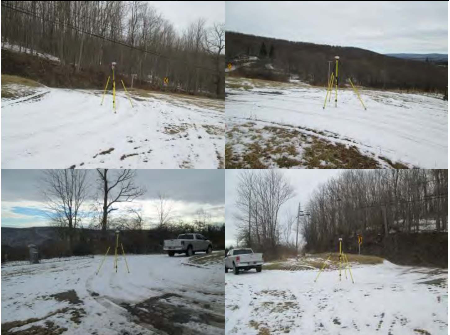
PHOTOS: Centerline of Drive @ Curve Midpoint
