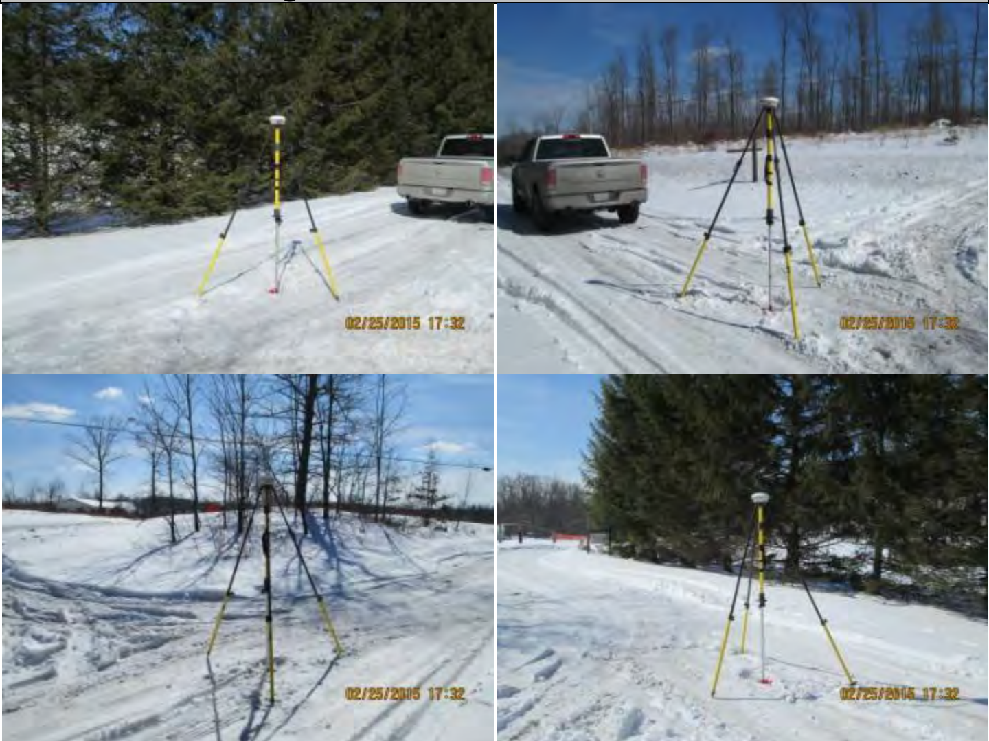
PHOTOS: Centerline of Road @ Centerline of Road
