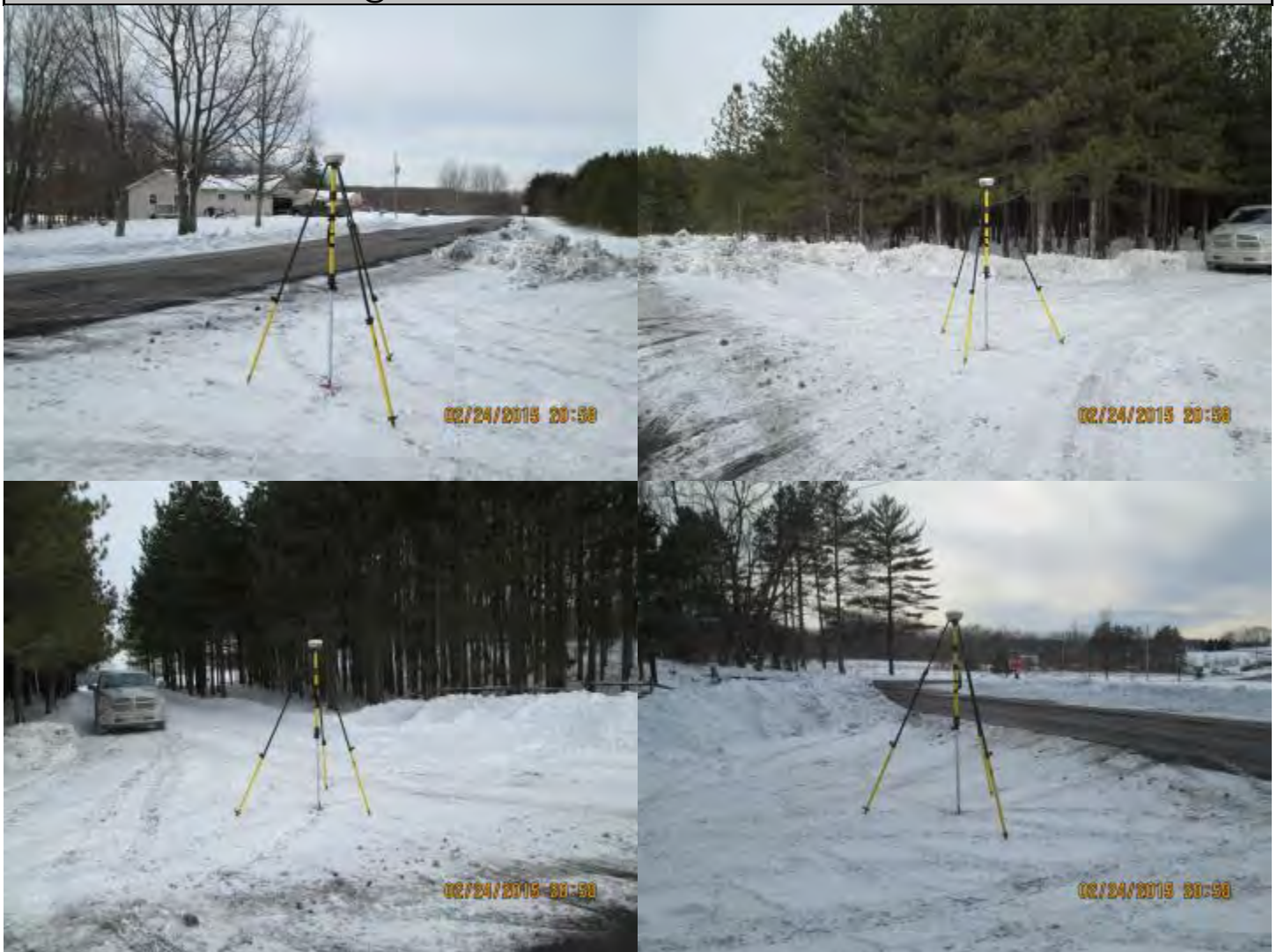
PHOTOS: Centerline of Drive @ Road
