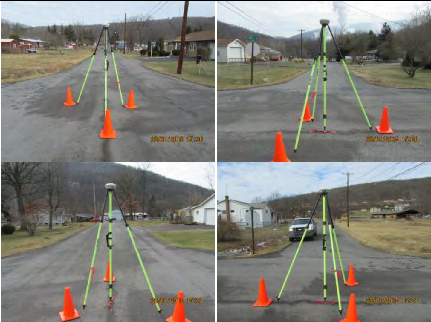
PHOTOS: Centerline of Road @ Centerline of Road
