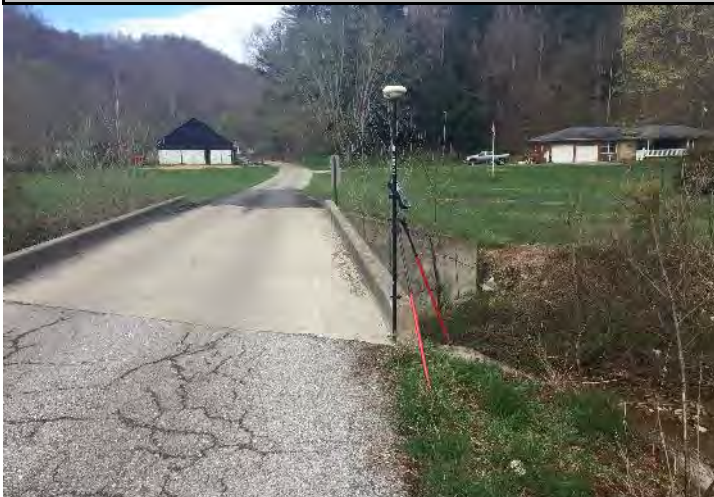
JD100 R033656 KY_Cal025 Pavement 2019-04-10 09:33:51-04:00 Quad: Vanceburg
