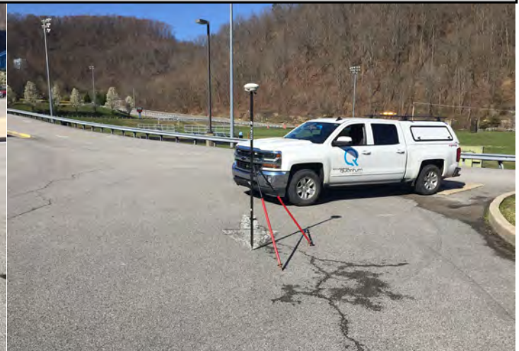
JD085 R033656 UA026 Pavement 2019-03-26 10:44:43-04:00 Quad: Elkhorn City
