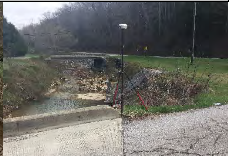
JD100 R033656 KY_Cal025 Pavement 2019-04-10 09:34:05-04:00 Quad: Vanceburg
