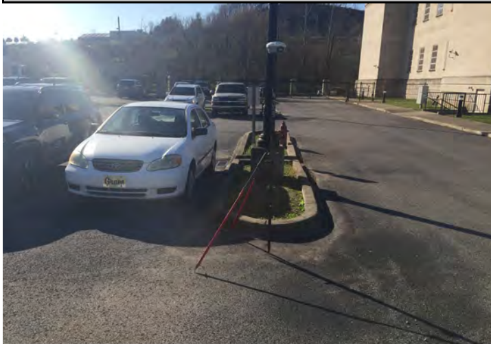
JD091 R033656 UA013 Pavement 2019-04-01 09:28:00-04:00 Quad: Paintsville
