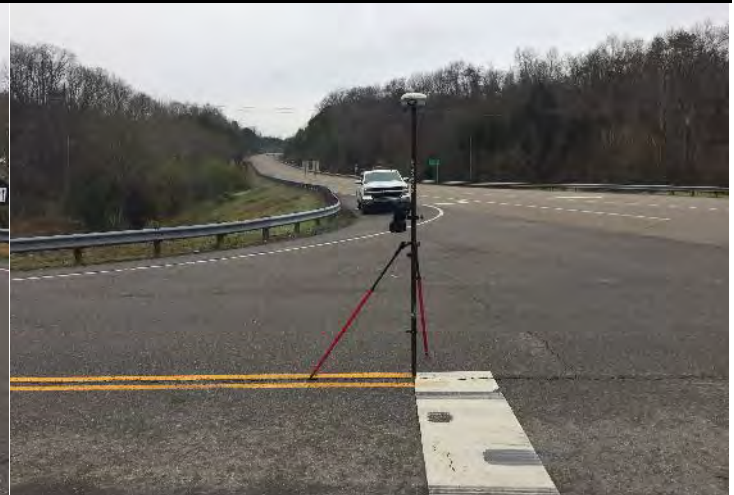
JD098 R033656 KY_Cal099 Pavement 2019-04-08 09:17:36-04:00 Quad: Load
