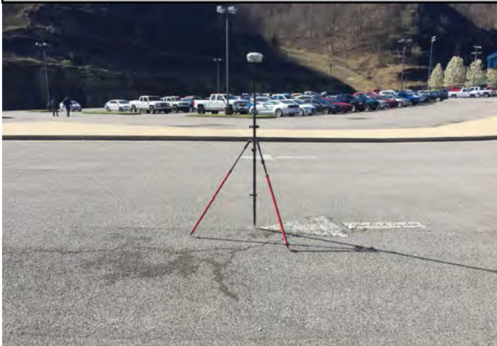
JD085 R033656 UA026 Pavement 2019-03-26 10:44:27-04:00 Quad: Elkhorn City
