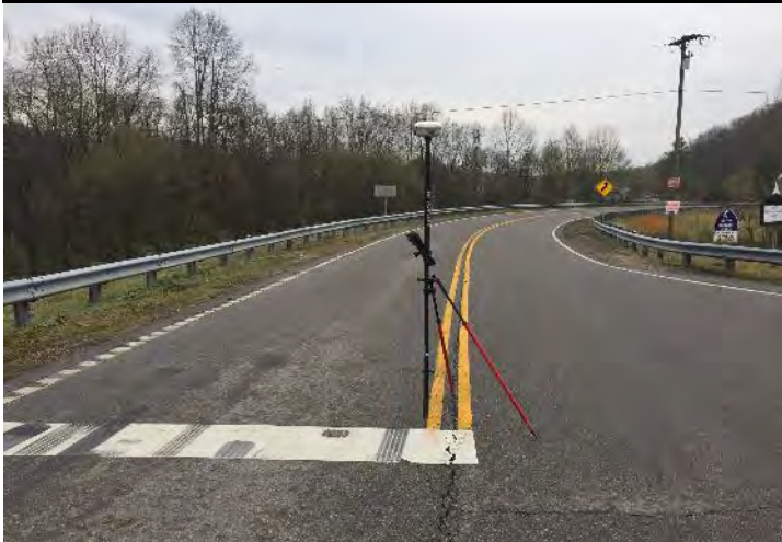
JD098 R033656 KY_Cal099 Pavement 2019-04-08 09:17:26-04:00 Quad: Load
