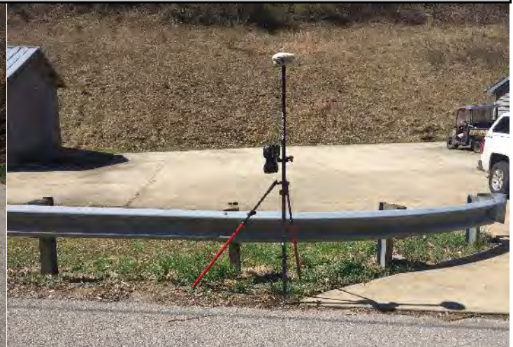
JD091 R033656 KY_Cal052 Pavement 2019-04-01 12:48:13-04:00 Quad: Oil Springs
