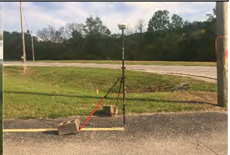
JD119 R033656 KY_Cal016 Pavement 2019-04-29 18:02:48-04:00 Quad: Maysville-West
