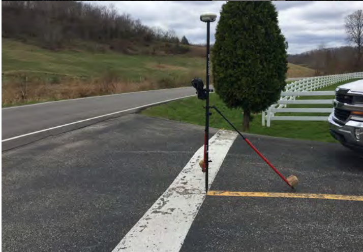
JD095 R033656 UA012 Pavement 2019-04-05 Quad: Fallsburg 12:59:23-04:00
